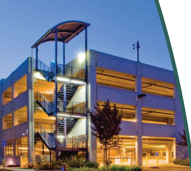
NEW GARAGE LIGHTING
