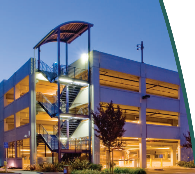
NEW GARAGE LIGHTING
